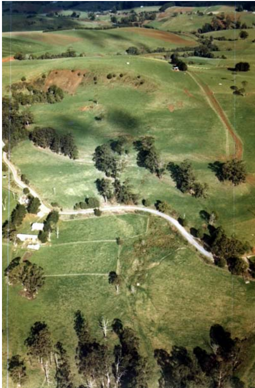
Figure 4.6 - Landslide No. 15 on the Trafalgar-Narracan Road, looking south onto a large landslide complex.
