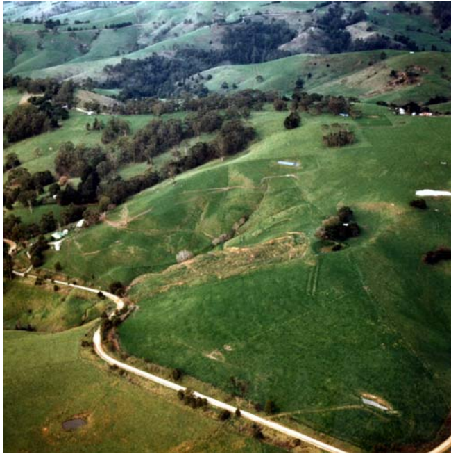
Figure 4.9 – Oblique aerial view of the Klevans landslide looking NE
