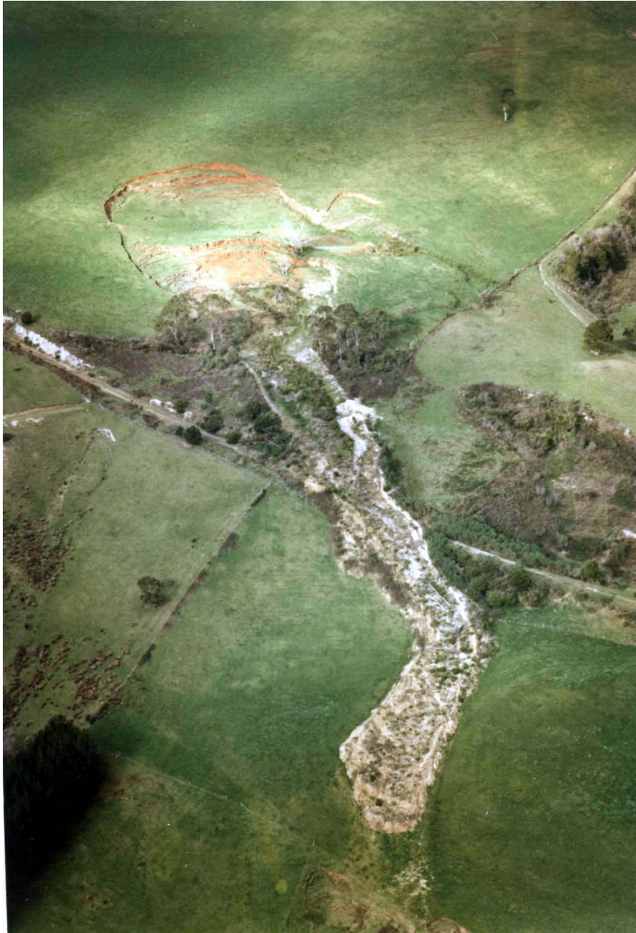
Figure 4.11 – Active slump-earth flow across Dingley Dell Road.
