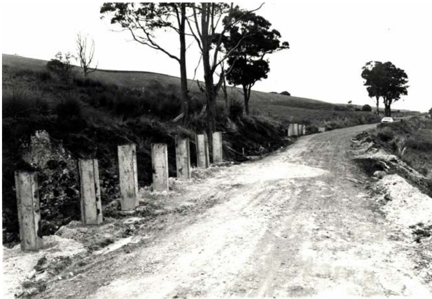
Figure 4.5 – Landslide No. 13, looking east along the Childers Settlement Road.
