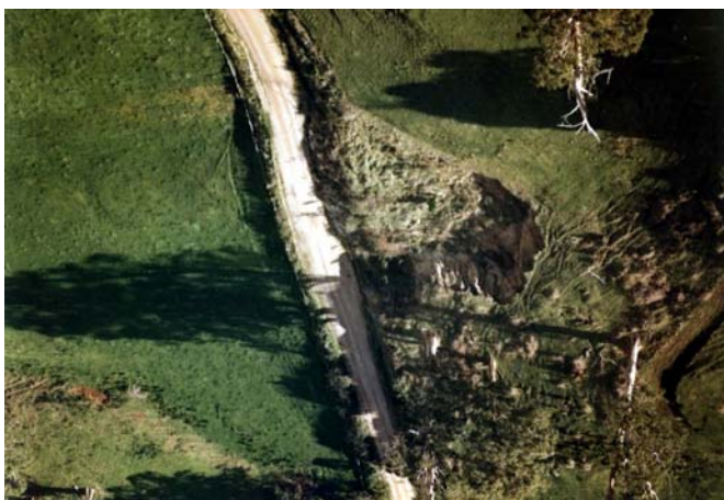
Figure 4.7 – Landslide No. 16, Trafalgar-Coalville Road
