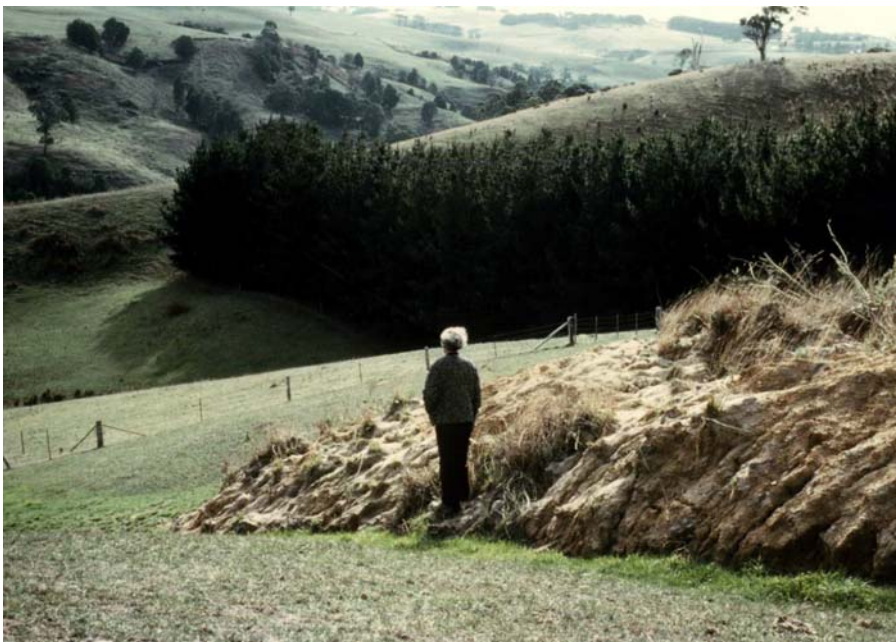
Figure 3.7 – Toe of earth flow zone of recent landslide, Dingley Dell. July 1978.
