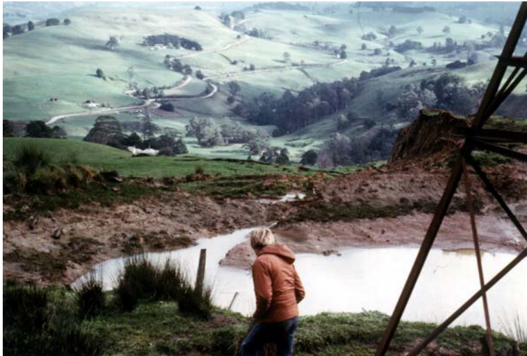
Figure 1.3 – Farm dam breached by landslide at Dingley Dell. July 1978.
