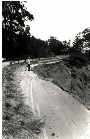
Figure 1.2 – Landslide in fill section of the main Trafalgar to Thorpdale road reduces width to one lane. April 1978.
