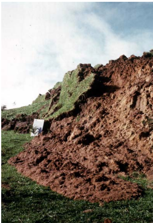
Figure 5.3 – Recent earth flow in friable, red-brown, silty clay of the Tertiary Older Volcanics. Dingley Dell landslide complex July 1978.
