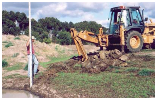
Figure 6. To reduce peak water flow run-off events, off-site buffer dams can be installed. Dam levels are kept low between rainfall events.
