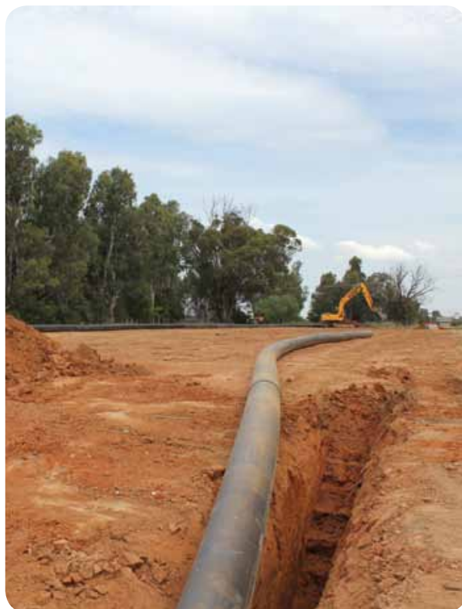
Pipeline being installed
