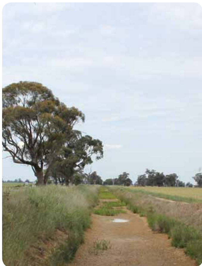
Open channel system
