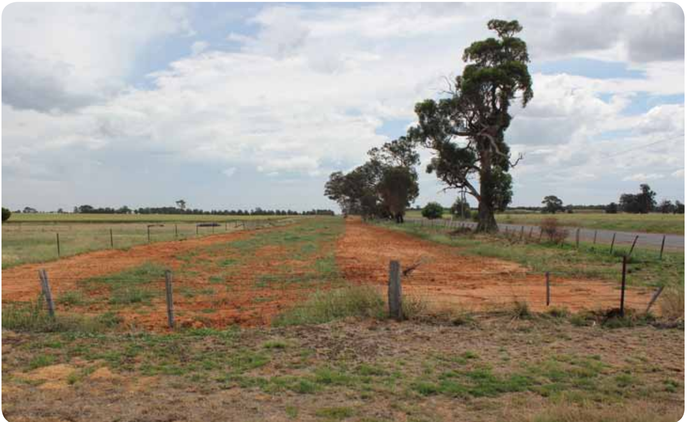
The completed pipeline installation
