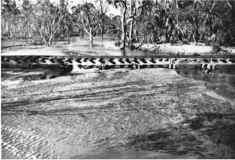
48. Siltation. Mokepilly Creek in Grampians, showing a bridge on the Stawell-Hall's Gap tramway, where 10 to 12 feet of silt have been deposited.
