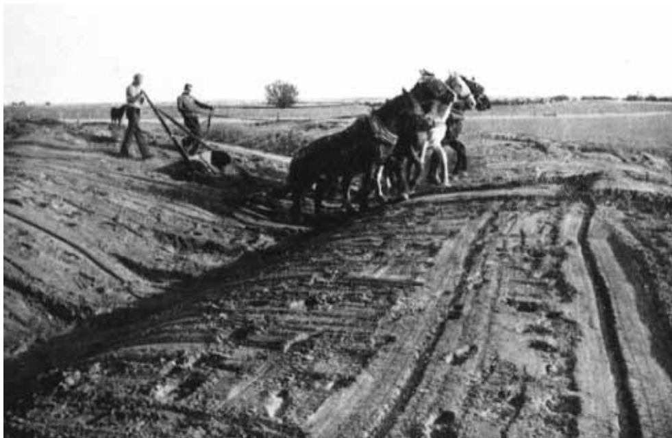
54. Scooping out channel shown in previous picture. Near Walpeup
