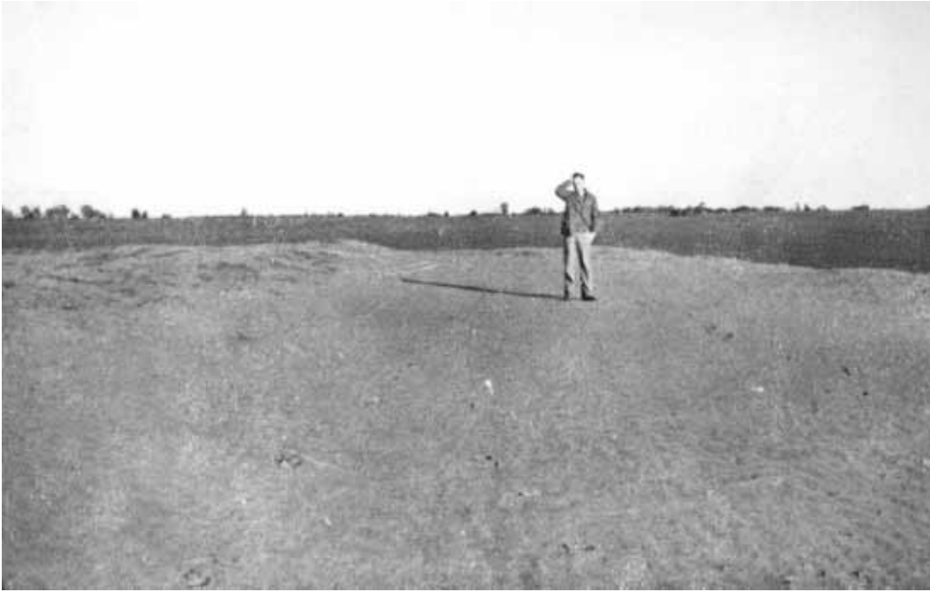
53. Main channel near Welpeup filled to the banks with drift sand from adjacent fallow.
