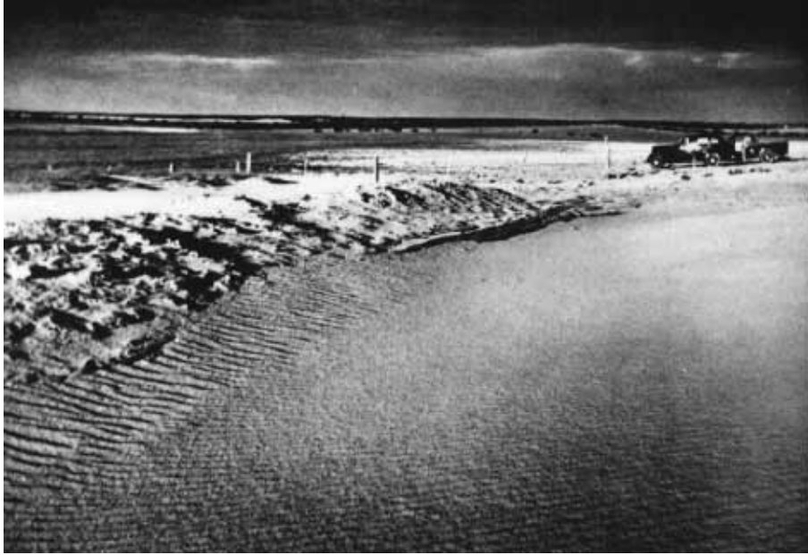
55. Parish of Kattyong - channel nearly filled with sand drift, only a few weeks after it had been cleaned out for use.
