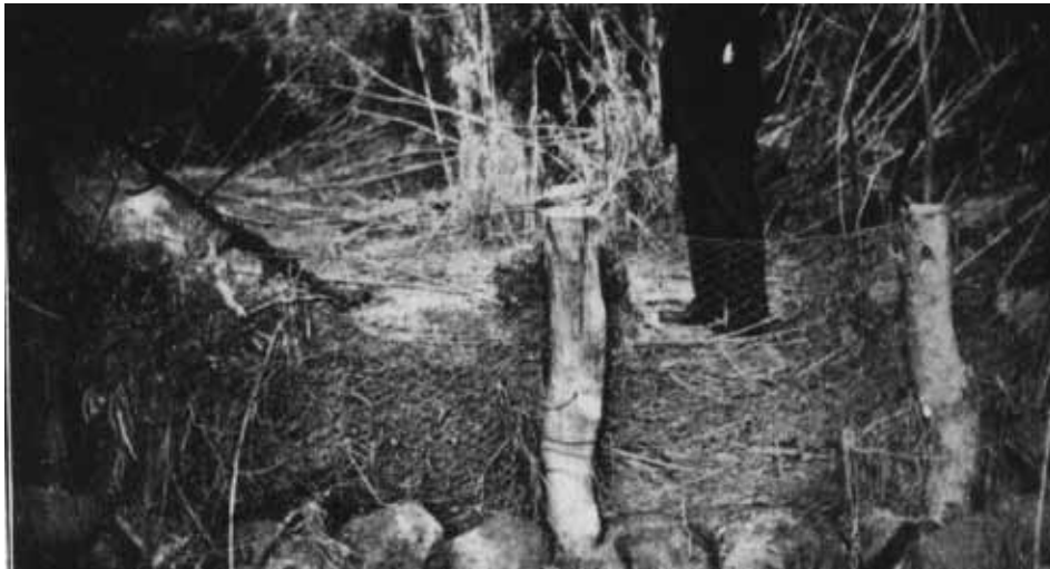
71. Showing how even ordinary wire netting will catch silt. Note how leaves, &c., have lodges against the netting, forming a silt trap.
