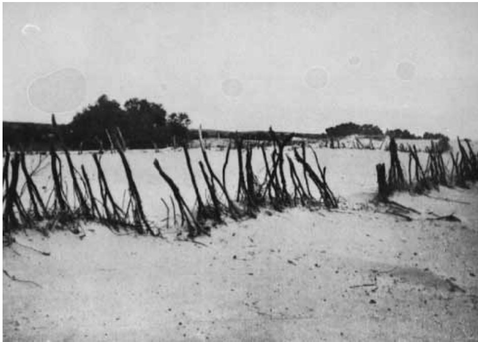
61. North of Hopetoun. Brush fence to check sand drift which was blocking channel.
