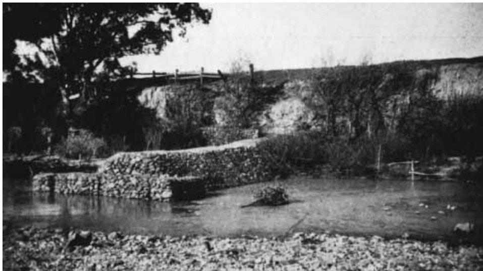
74. Lerderberg River, Bacchus Marsh. Protection of eroding bank. Shingle and wire type groyne, showing siltation to original end of groyne in two years, and recent extension. Note willow stakes in silt bench.
