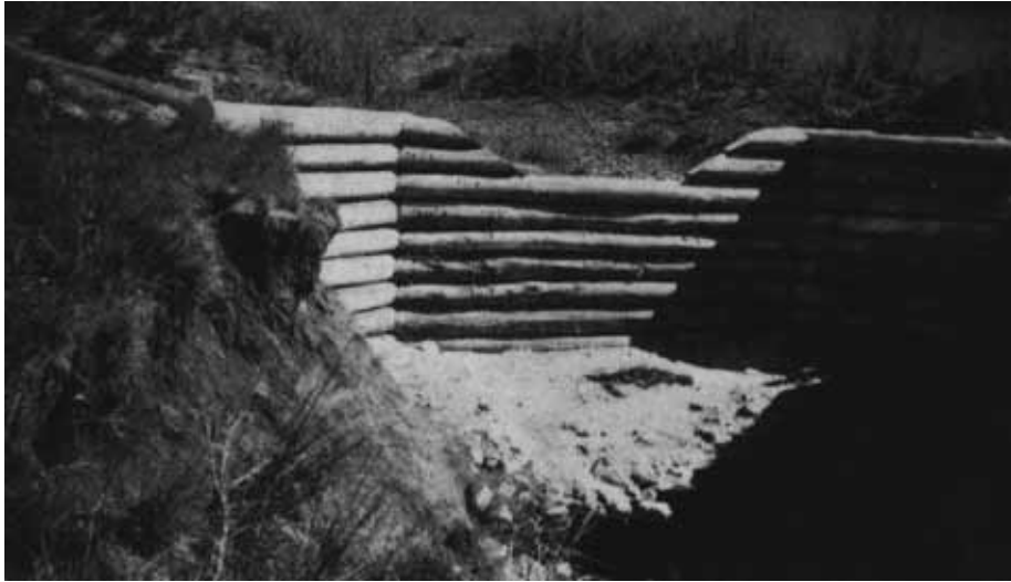
64. Log dam across scour near Bindi Station. This is now filled to the top
