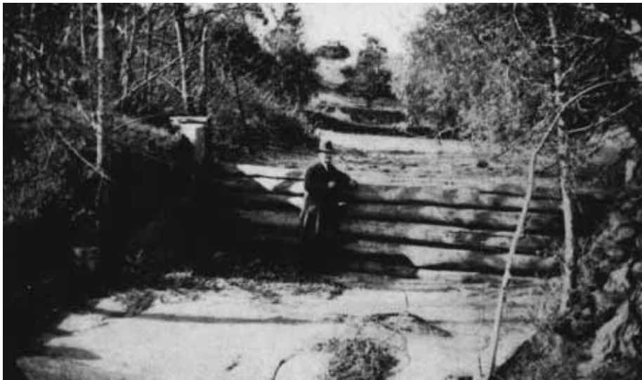
65. Check dam to stop scour alongside Gisborne road, Bacchus Marsh Shire
