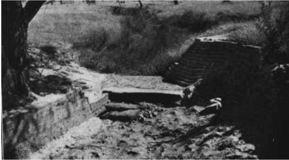
70. Near Benalla. Brick and concrete drop constructed by land holder in scouring gully. This has been effective in preventing extension of scour.
