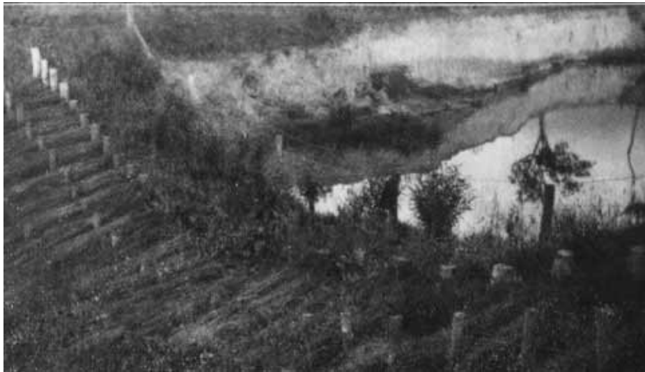
68. Brush dam to catch silt derived from eroding banks, Skull Creek, near Bairnsdale.
