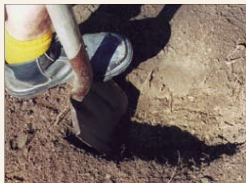
Figure 1 Dig a hole 50-60 cm deep.
