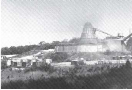
A timber mill near Woodend, which processes mainly native hardwoods from the adjacent State Forest.
