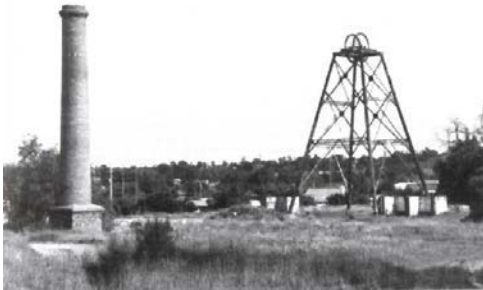
Evidence of gold-mining days can still be found throughout the catchment, such as this poppet head and chimney stack at Bendigo
