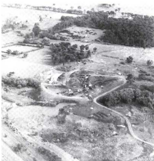
A road-metal quarry near Tylden
