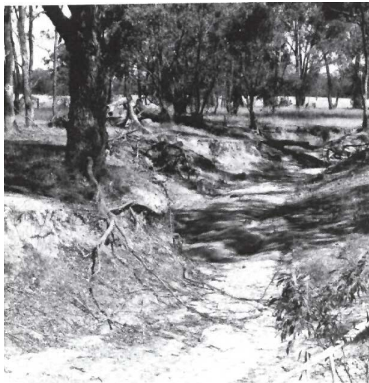
Increased run-off has scoured the drainage depressions and transported large quantities of sand into Mount Pleasant Creek.
