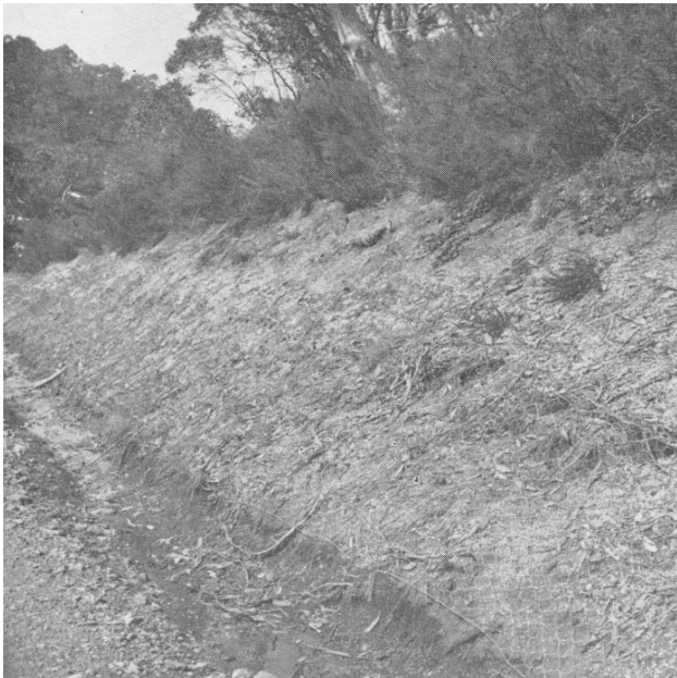
Plate 21. A road batter on which seed and fertiliser were applied and covered with a mulch of hay held in place with wire netting. The mulch has rotted. Establishment of vegetative cover is not satisfactory.
