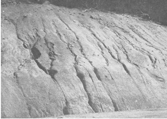
Plate 20. The bare eroding batter of the recently (1968) enlarged vehicle park at Dingo Dell.
