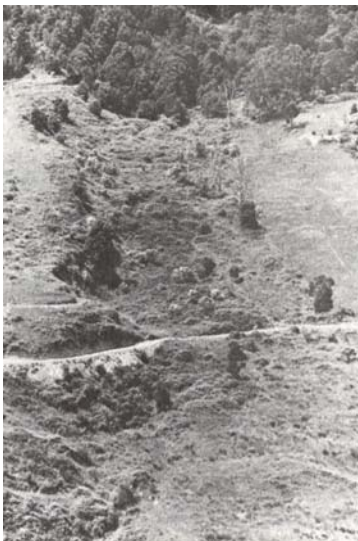
Earth flows are a common feature of the steep hills: This one near Upper Gellibrand threatens the road that crosses it.
