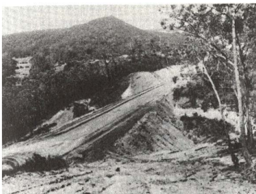
Large road batters and other bare surfaces can deteriorate rapidly. This road re-alignment near Mount Mackenzie is a source of copious sediment in the Gellibrand water supply catchment.
