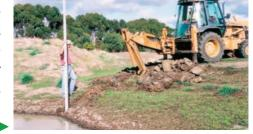
The above system has been extended to include a buffer dam. On a flat headland, an underground collector pipe has been installed with a predetermined fall to the dam. For this system to work, the level of the dam must be kept below the inlet pipe.
