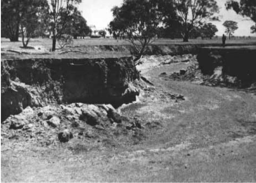
27. Bullock Creek, north of Marong. The debris from this has silted up the creek lower down blocking bridge and increasing flooding problems on the flatter land.
