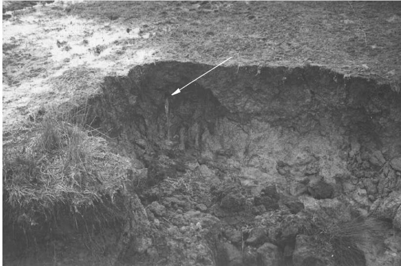
Plate 15. Tunnels formed in valley marsh soil.
