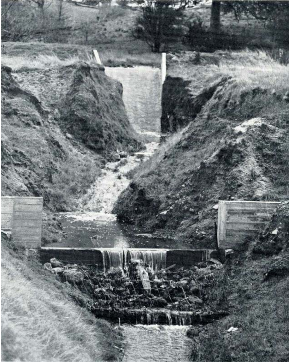
Two concrete structures solve a difficult gully erosion problem.
