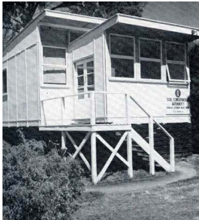
The office which was built at Heathcote is the centre for operations for the project. Behind the office there is a large storeyard, sheds and a tree nursery.
