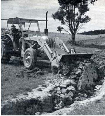
Filling in a small gully which will become unnoticeable when the paddock is chisel-seeded and sown to improved pasture.
