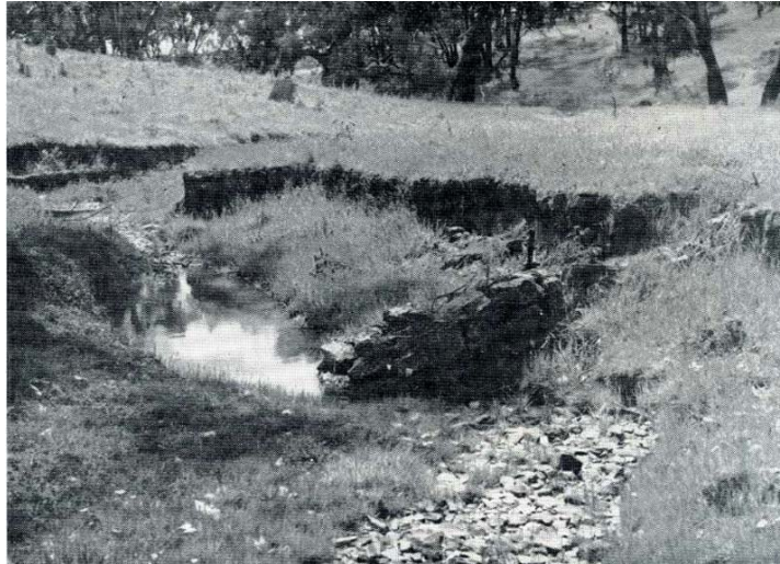
The healing effect of soil conservation works in the paddock is shown in this gully which is no longer eroding.
