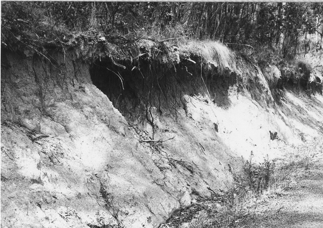
Mountains on gneiss: Road cutting showing shallow soil on weathered rock that is typical of steep slopes with dry forest in this land type.
