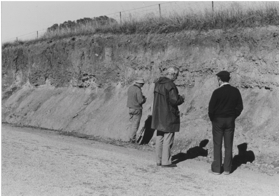
Low hills and undulating terrain on schist, sedimentary rock and derived colluvium and alluvium: Road cutting along Georges Creek road showing an inspection of unconsolidated material of different depositional phases/and soil development.
