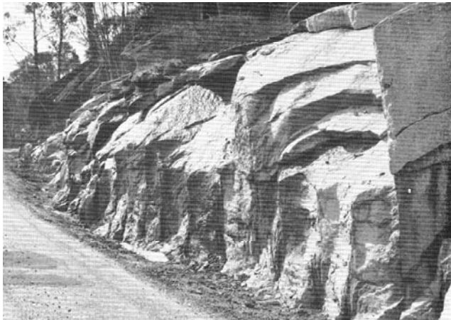
Plate 2 – Exfoliation layers exposed by a road cutting. Exfoliation (scaling off of rock in layers) is an important form of weathering in granite.
