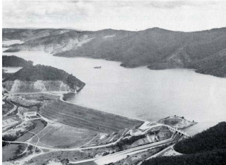
Plate 2 – Lake Eildon has been formed by the construction of an earth and rock dam
