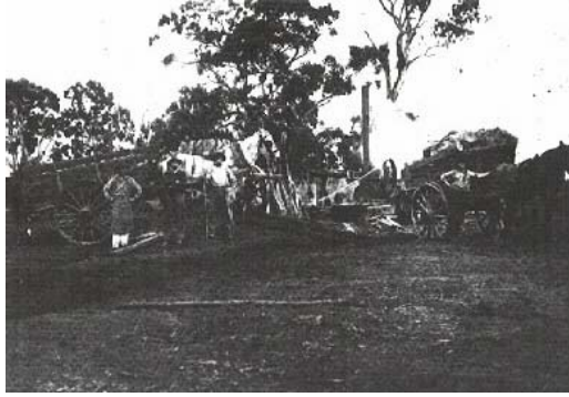
Plate 2.6 On-site mill for cutting firewood near Seymour (circa 1903). Seymour Historical Society.
