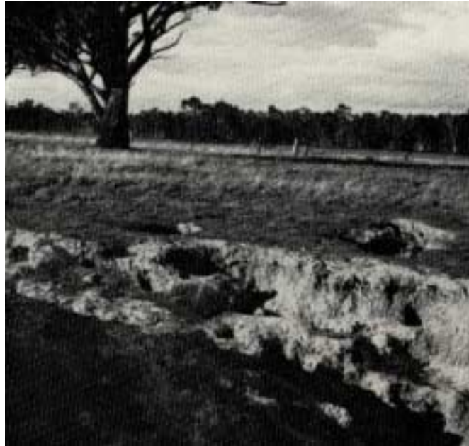
Plate 32. Tunnel erosion is commonly associated with yellowish duplex soils. In this example the tunnels are in various stages of collapse. They lead into the gully system shown in Plate 33.
