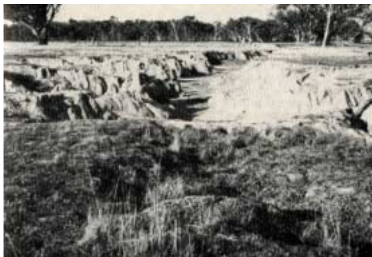
Plate 33. A gully system which has formed from collapse and coalescence of numerous erosion tunnels. The water of Lake Mokoan is just beyond the fence in the background.
