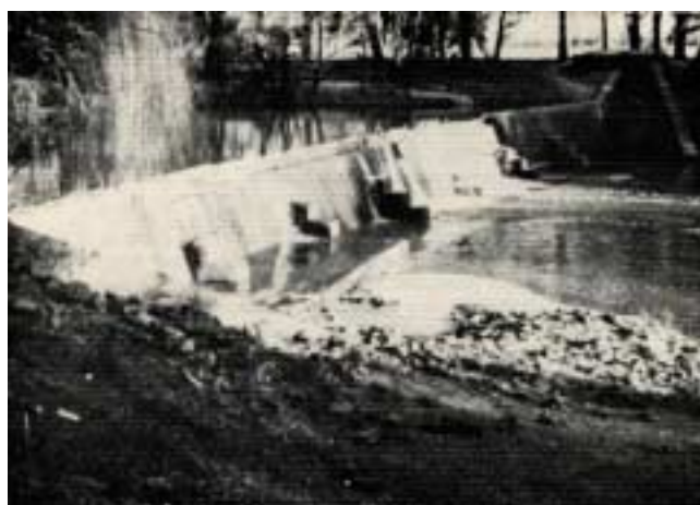
Plate 2, Casey's Weir on the Broken River at Goorambat allows water to be diverted to the north for stock and domestic purposes.
