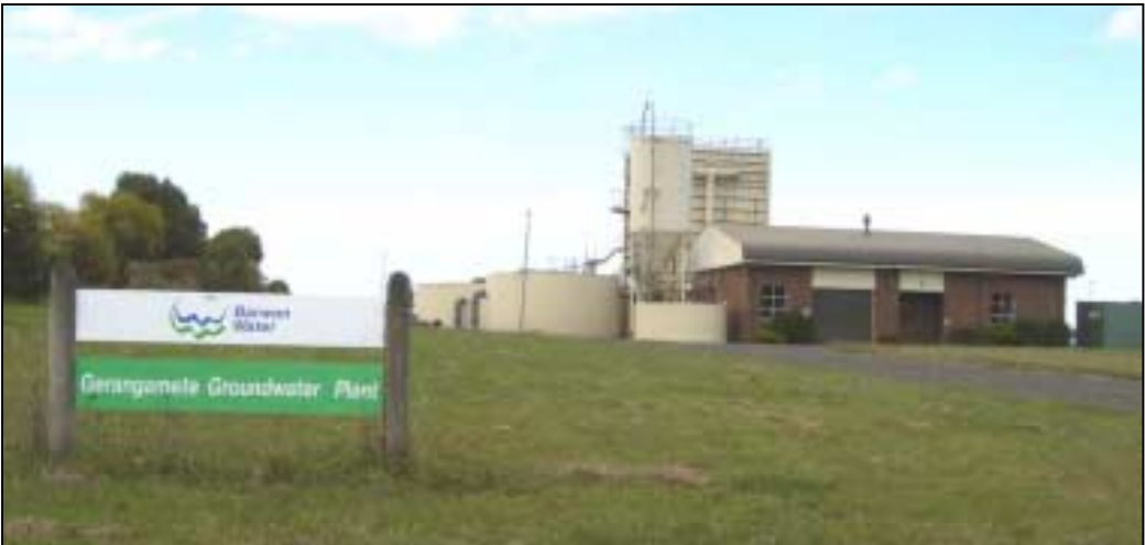
Groundwater Station at Gerangamete supplements Geelong's water supply.
