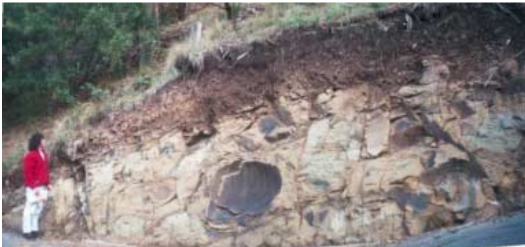
Cutting showing fractured sandstone and soil cover at Morley Avenue, Wye River
