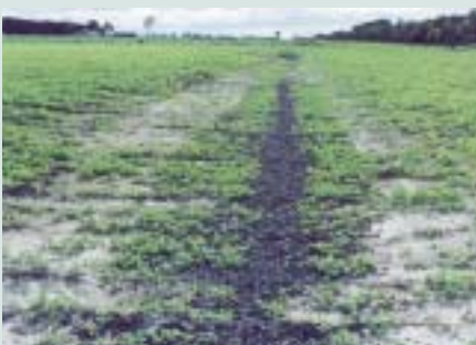
The underground treatment in late winter. Note the slightly wet areas between the gravel and the beds in the foreground. This apron had a slope of approximately 1%.
