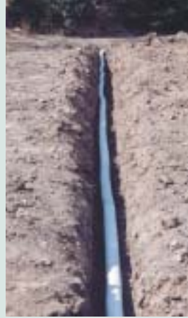
To relieve the drainage water from each treatment, a drainage pipe was taken across the headland to the fence line.
