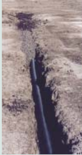
The 100mm slotted agricultural drainage pipe laid in the trench.
