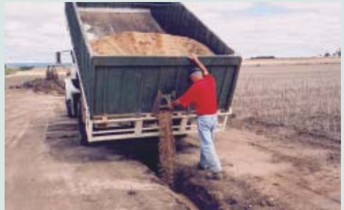
This season we became mechanised. Here the farmer's grain truck was used to add the gravel base.
