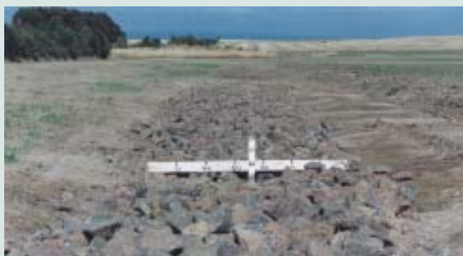
One of the finished large crushed rock treatments.
