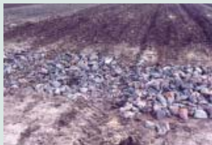
The large crushed rock treatment took the weight of the machine but the rocks squashed into the mud. The tractor driver said he needed to slow down to cross the collector drains. He was also worried about potential damage to the tractor tyres.
