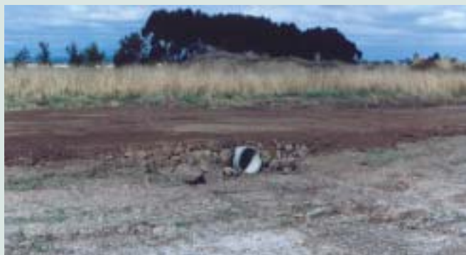
Culverts at lowest point in paddock
