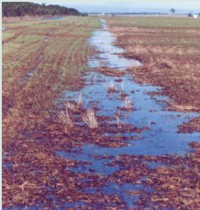
Poorly drained collector drain
