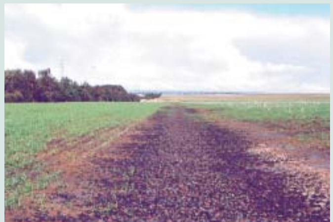
This is the same collector drain shown on page 2, again after approximately 50mm of rain.
