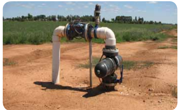
In field secondary filter and control valve
