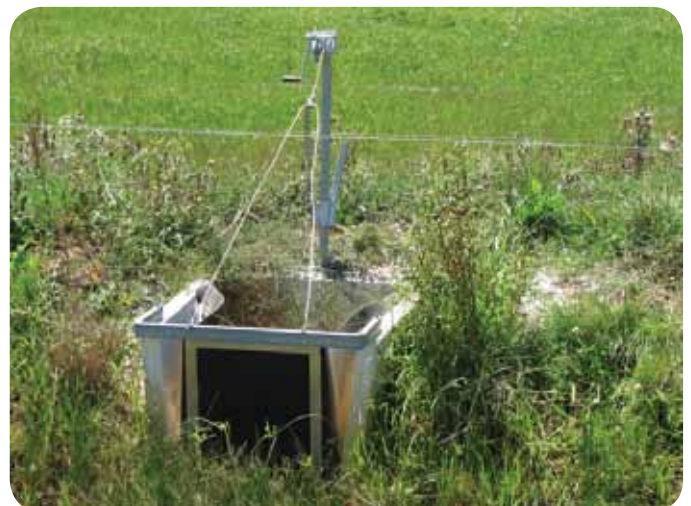
High flow piped Padman bay outlet
