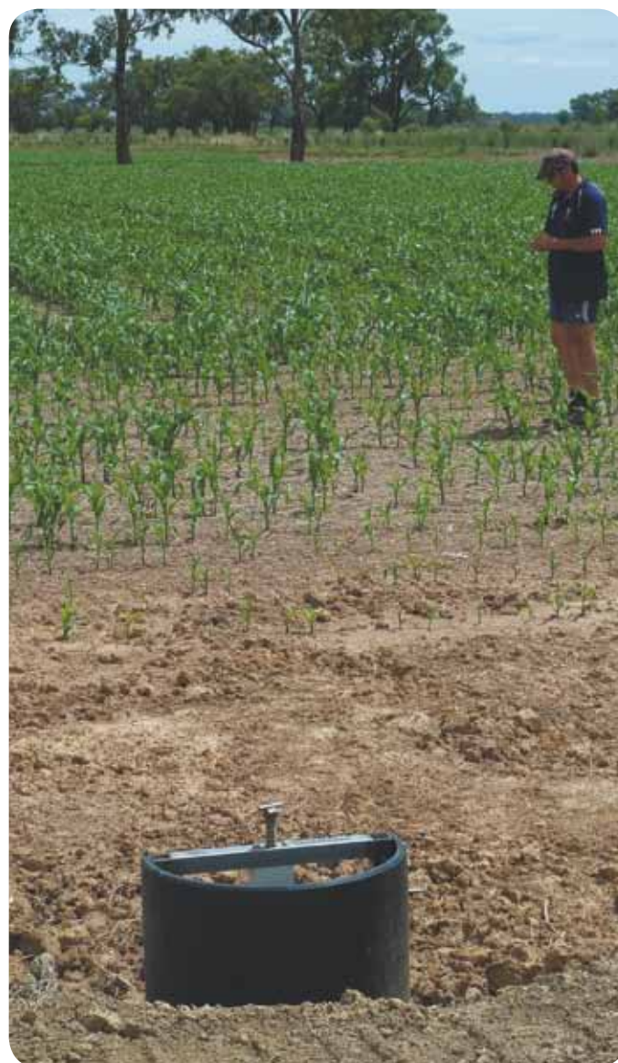
Pipes and Risers: Brad near his farm's pipe and riser system
