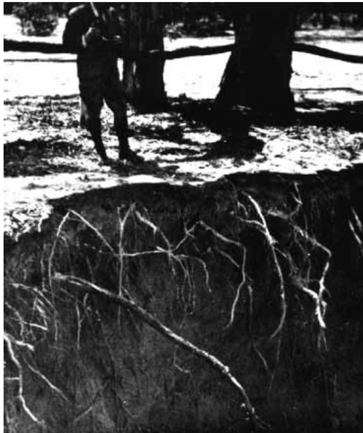
17. Head of deep scour, about half a mile long, near Toolern Vale. This is said to have started from a furrow run down a slope to lead water to a dam. It is now 15 feet deep, and has invaded a road.
