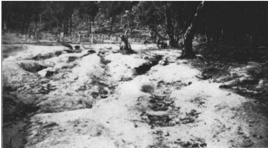
19. A road in granite country, north-east of Wangaratta. The surface has been stripped off by traffic, and gulying has commenced.
