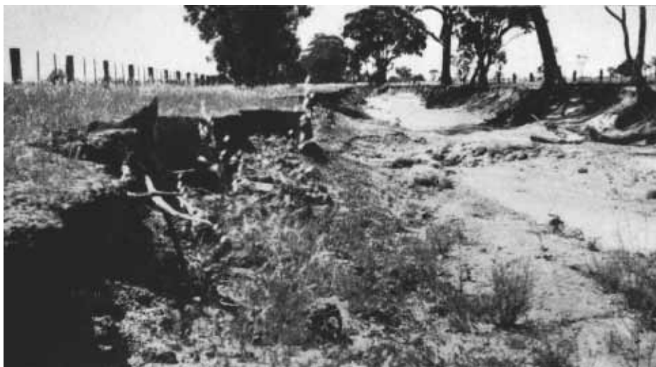
26. Spring Creek comes down from the hill west of Bendigo, and used to spread over the flatter land near Derby. A drain was cut down a road, perhaps 40 years ago, to continue the waters of the creek. This has scoured till it now occupies nearly all the road.
