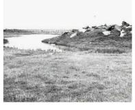
Bedrock is usually close to the surface, as indicated by the basaltic boulders in the excavated dam-bank material.
