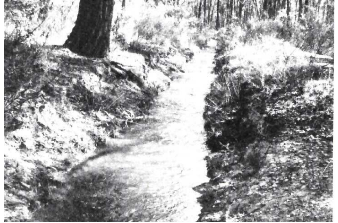
Open channels convey water to private properties
