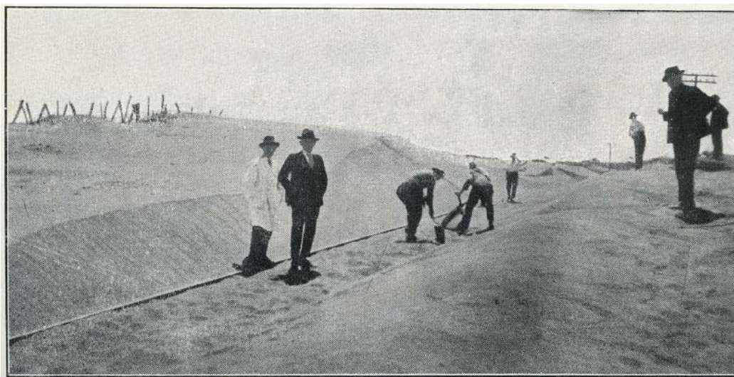
Mittyack Railway Line showing sand hill encroaching on line
