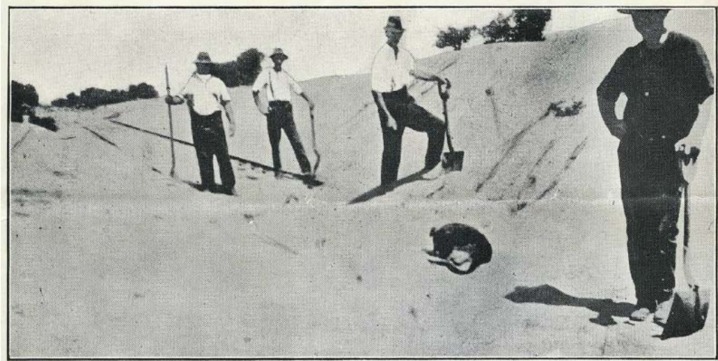
Patchewollock Railway Line showing both rails covered with sand
