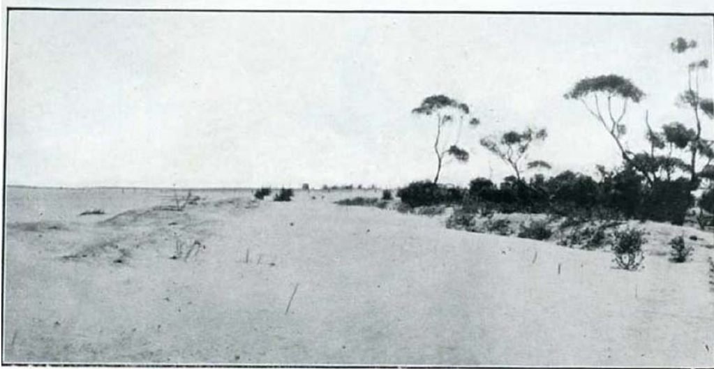
Main Channel near Woomelang completely blocked by drift from fallow. Note that there are no sandhills near the channel.
