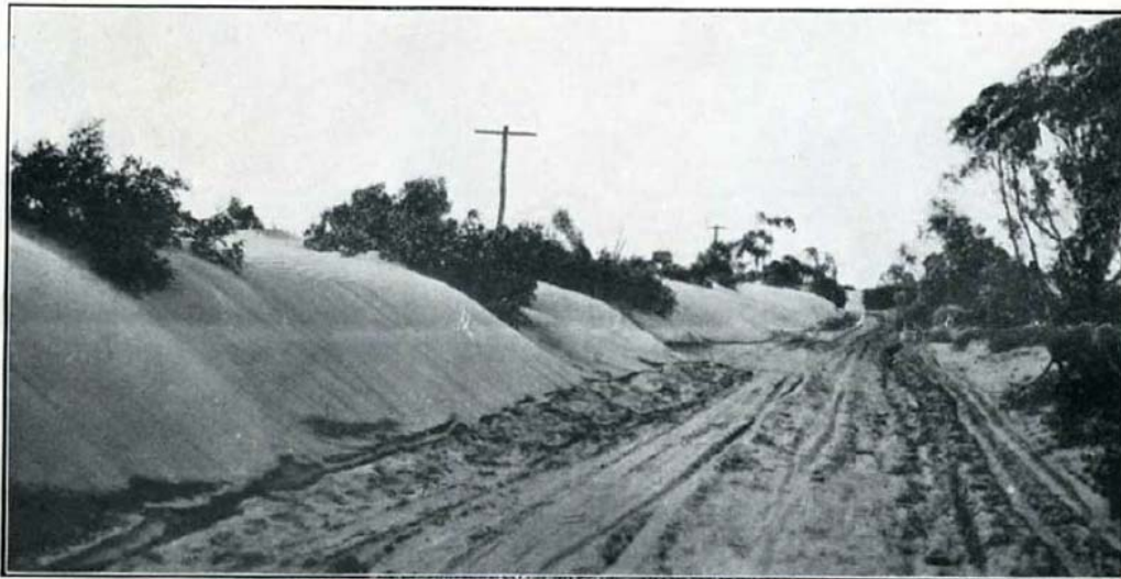
Road, Walpeup – Sand drift from fallow has smothered the Mallee scrub, and is fast encroaching on to track
