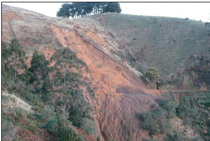
Figure 2. Landslide on Wild Dog Creek Road, 1979.
