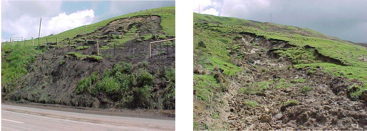
Figure 3. Two adjacent landslides that impacted on the Great Ocean Road, October 2000.
