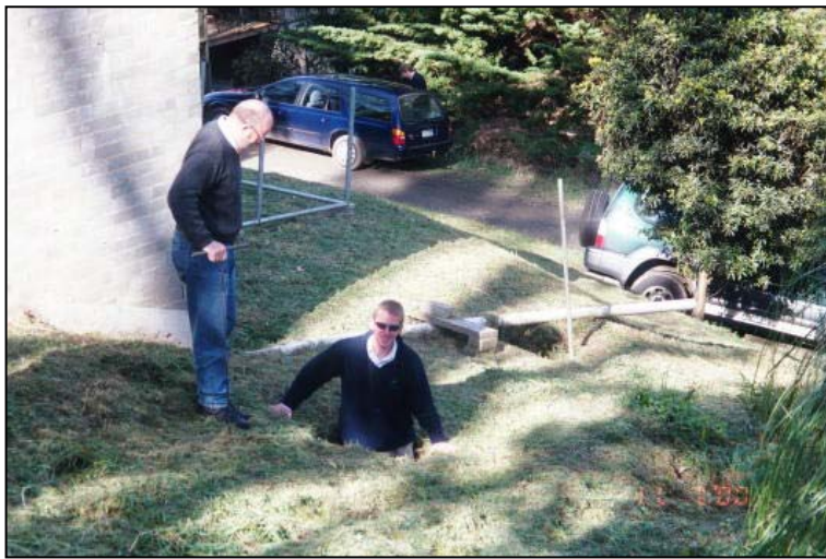
Figure 3.2 Tunnel erosion adjacent to a house in Separation Creek.
