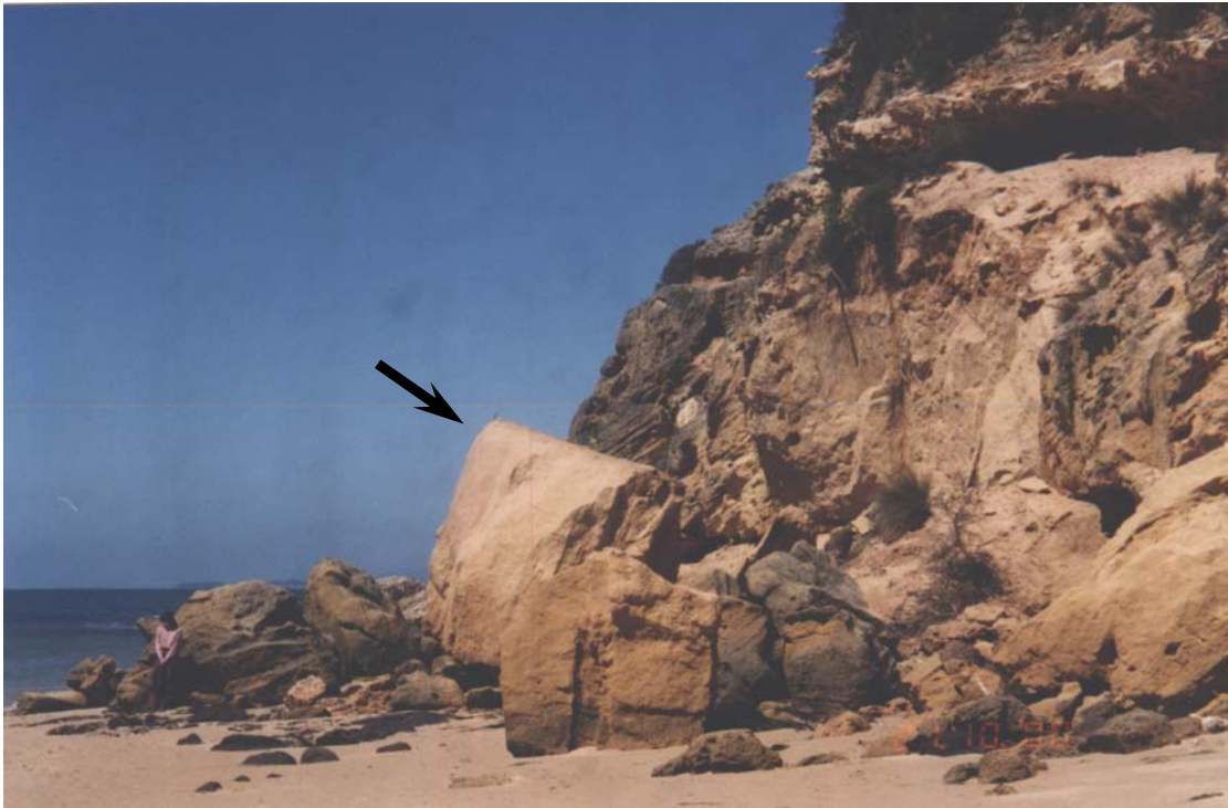
Figure 2.2 An example of a rock fall at The Bluff, Barwon Heads.
