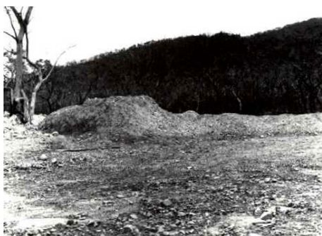
Shallow excavation: Minor gravel stripping from the lower rocky colluvial slopes (Qrc), of the well vegetated Sedimentary sandstone formations (Clk)
