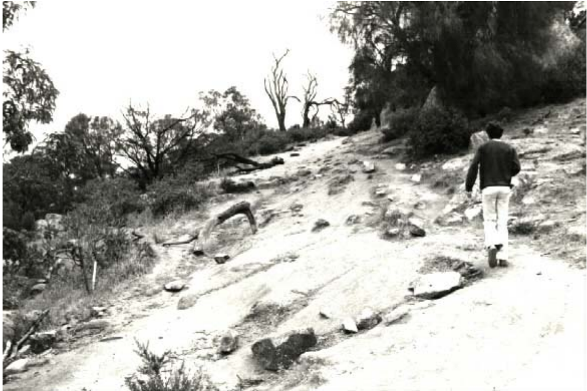
Plate 5 – The existing walking track to Flinders Peak is ill-defined, devoid of vegetation and badly eroded.
