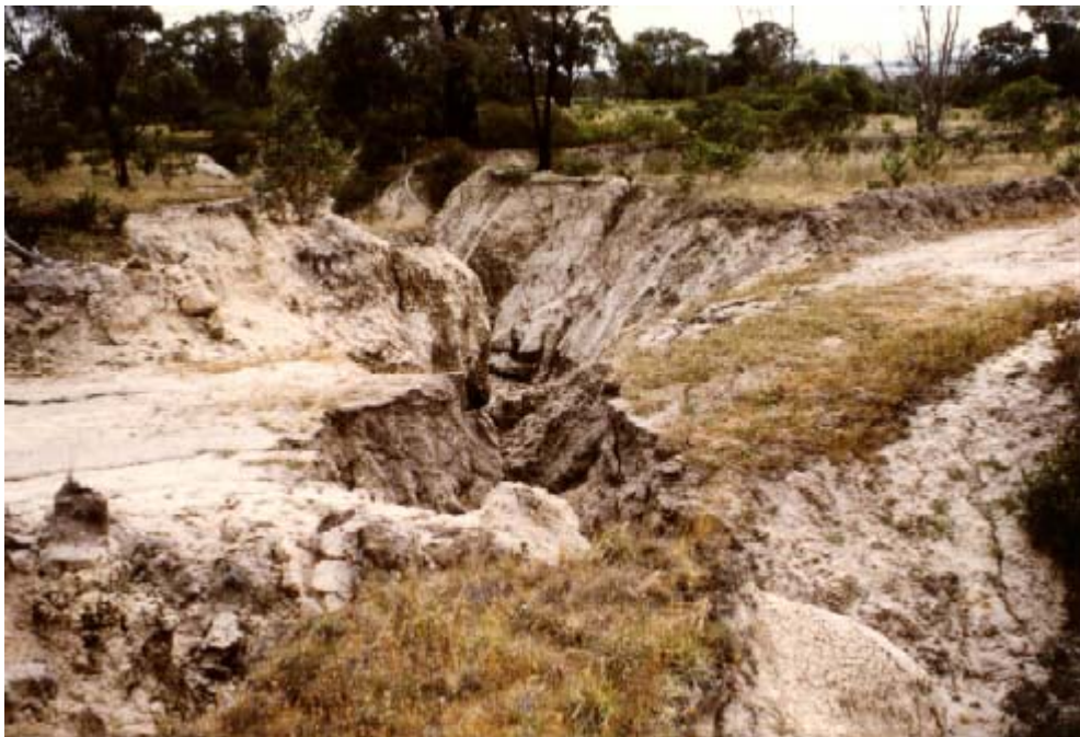
Plate 4 – Severe gully erosion running through the reserve has been initiated by sand scraping operations in adjacent areas
