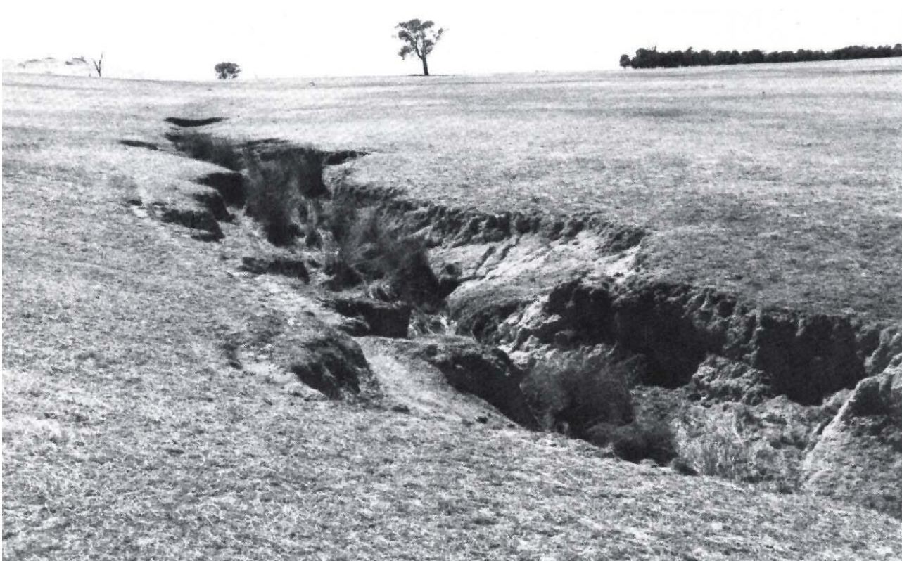
Gully erosion, although not severe, is common
