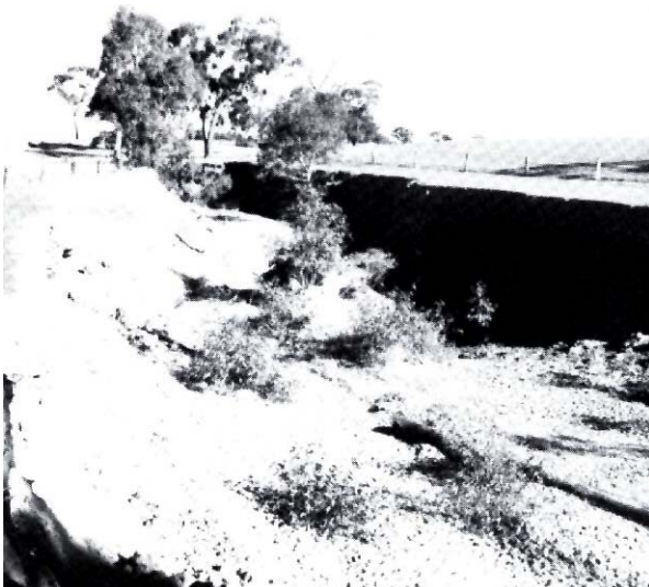
Severe gully erosion occurs when excessive run-off from adjacent sloping land is channelled into these gentle drainage depressions.
