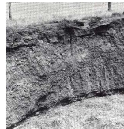
The ridge of sandy material along the fence-line indicates the extent of wind erosion over the years.
