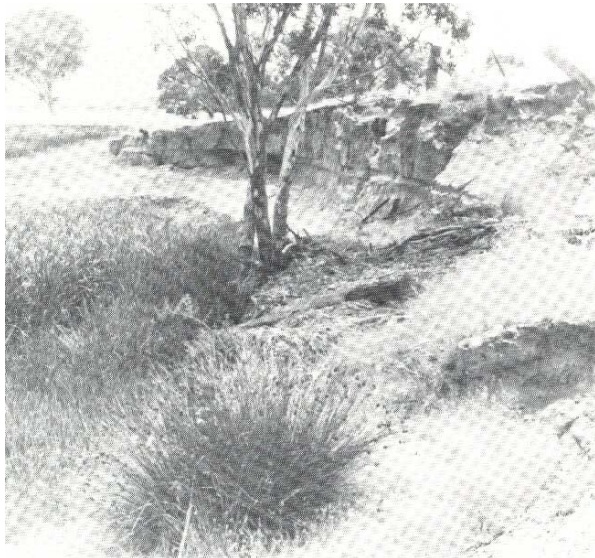
Streambank erosion (above) is an active process during flood periods.
