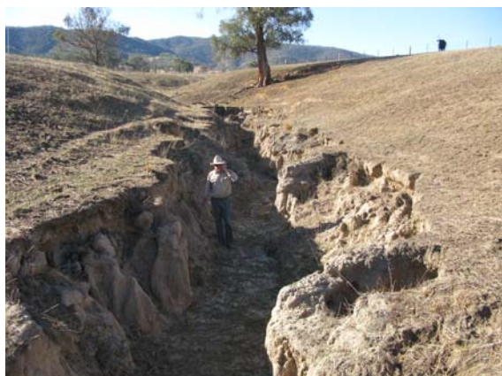
Figure 1: Before rock chute
